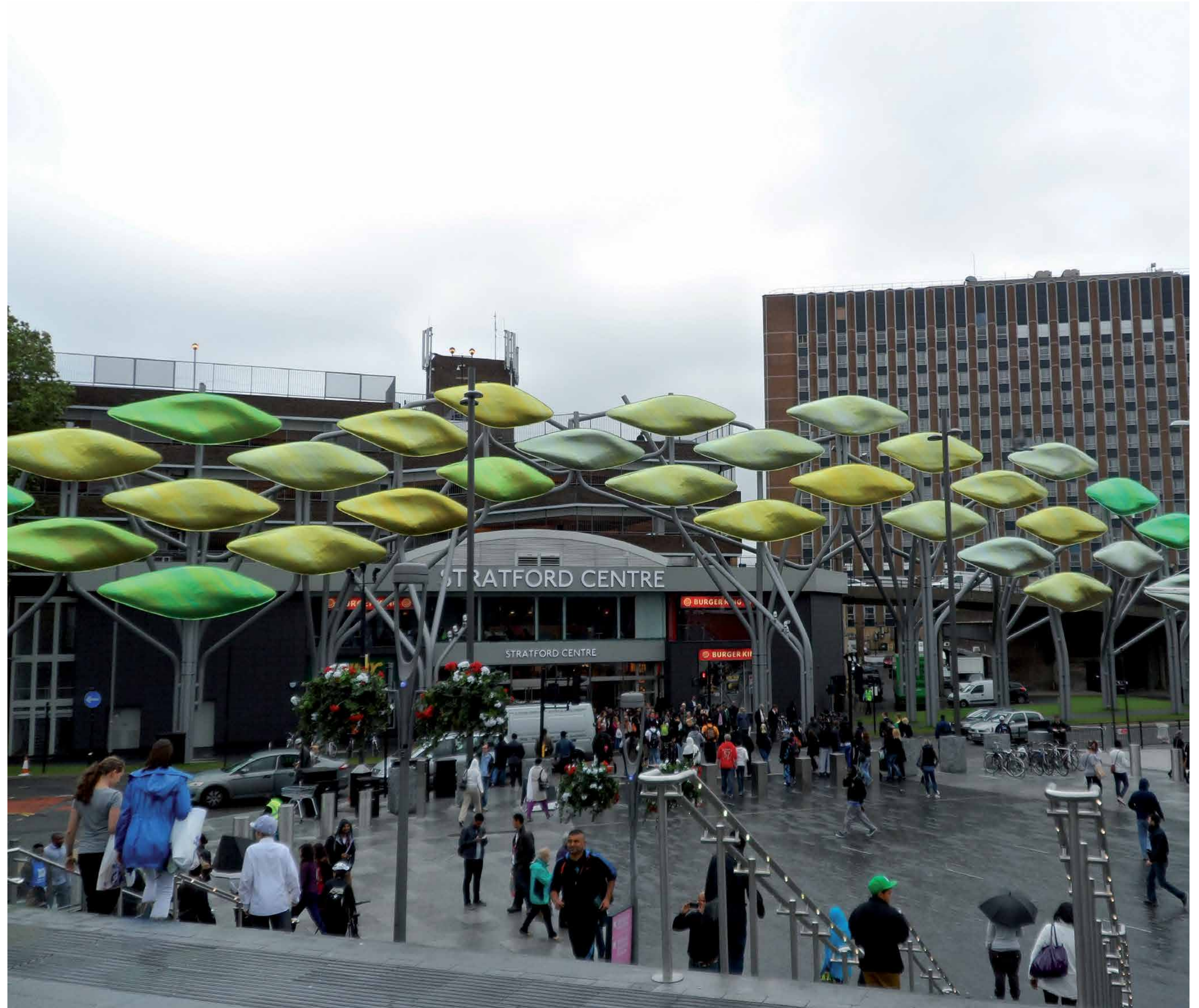
A photograph of the front of the Stratford Centre as it currently appears
