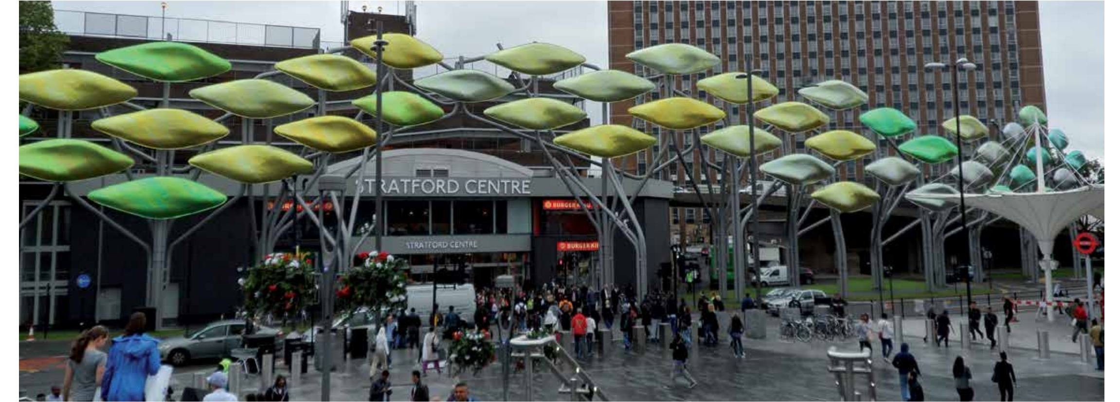
A photograph showing Morgan House and the Stratford Centre
