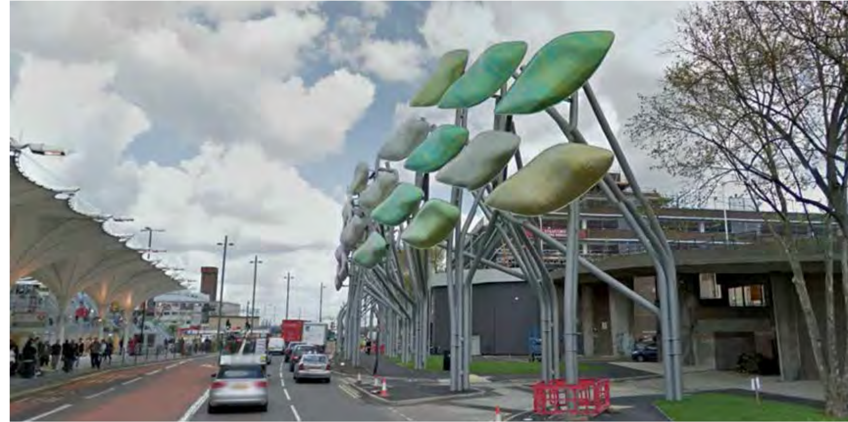
A photograph of the public realm along Great Eastern Road
